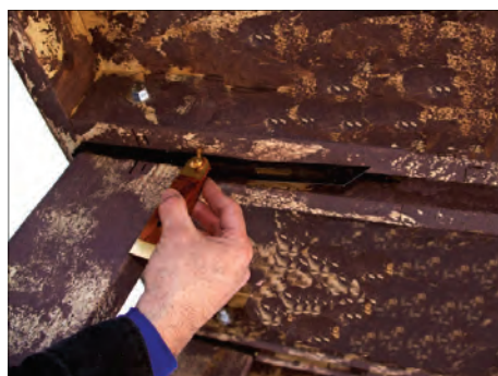
Photo 3 - Check the angle
