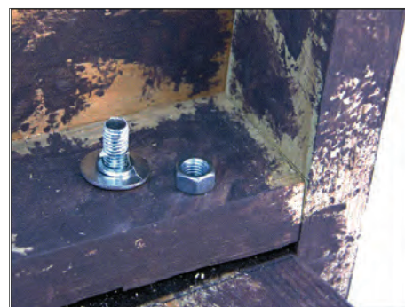
Photo 6 - Install 1/2" Flat Washer, Lock Washer and Hex Nut. Tighten securely.
