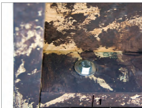
Photo 5 - Install 1/2" Hex Bolt with Flat Washer
