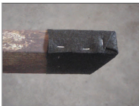
Photo 2 - Install Landscape Felt
