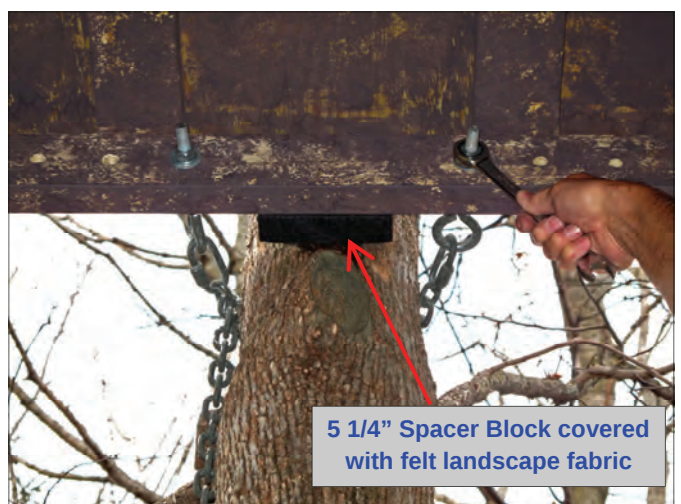
Photo 4 - Tighten Hex Nuts
