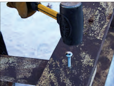
Photo 4 - Drill 3/8" Holes, Install 3/8" Carriage Bolts, Flat Washer, Lock Washers, and Hex Nuts. Tighten securely.
