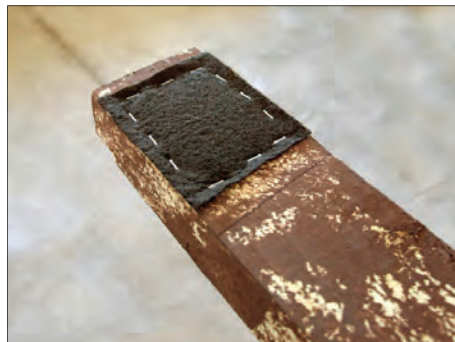
Photo 2 - Install Landscape Felt
