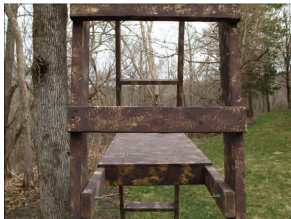
End View of Lower Platform Installed on Stand
