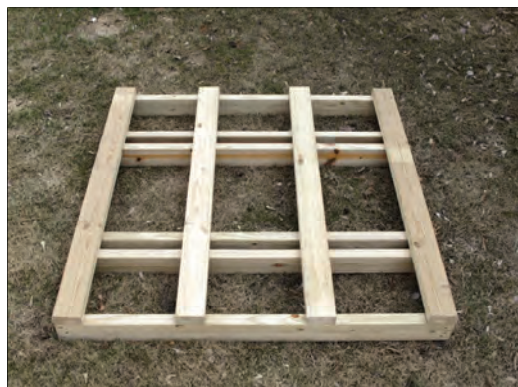
Completed Upper Platform Frame
